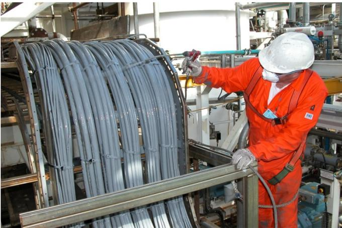
**Avicoat** is often used in confined spaces in underground and marine / shipping situations where burning cables can create hazards from smoke, toxicity and unnecessary power failure.
