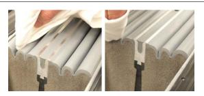
Prior to installation, this release agent must be wiped off all surfaces that will later make contact with liquid applied silicone. This includes, the face, tops and grooves of the bellows next to the face, and along the sides.
